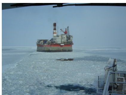
Figure 4.6: Broken ice in the wake of a platform
